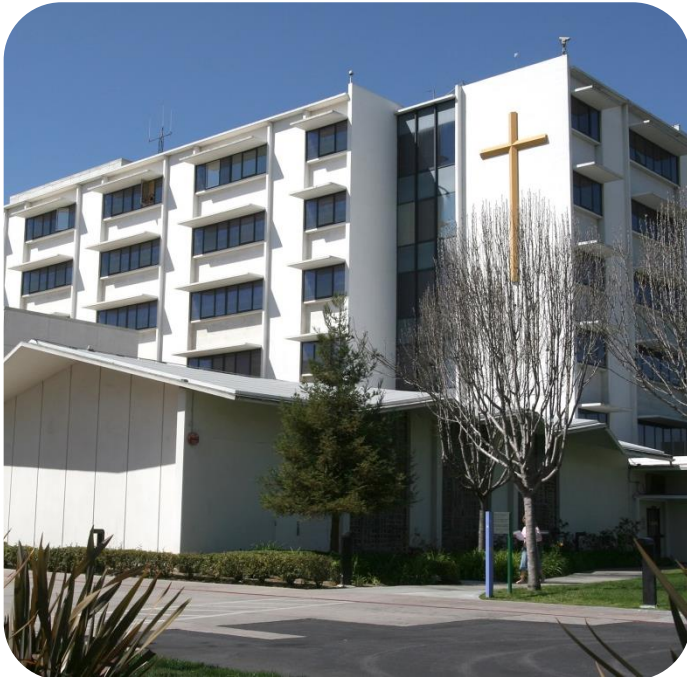
Queen of the Valley Hospital West Covina
